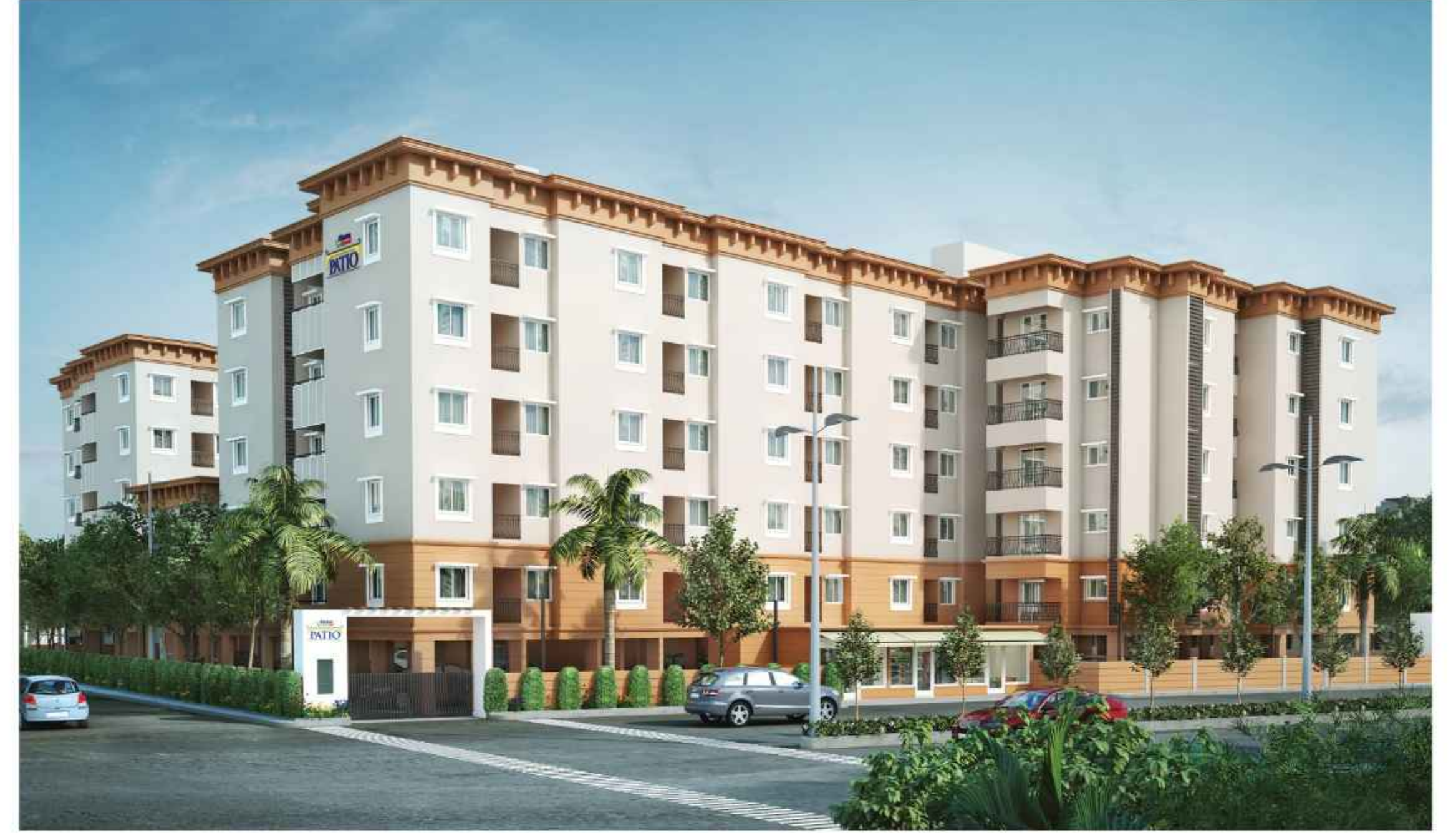
PATIO – 157 Units, Neelambur, Avinashi Road, Coimbatore.
